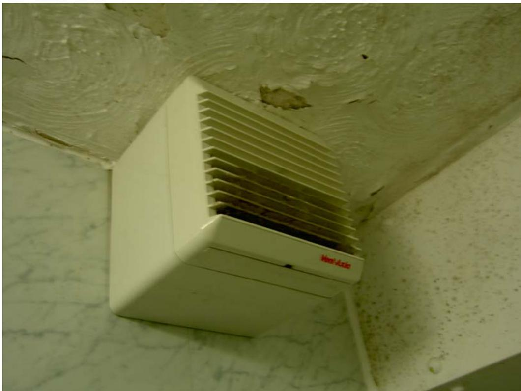
Figure 6.3c—Vent duct connected to outside
