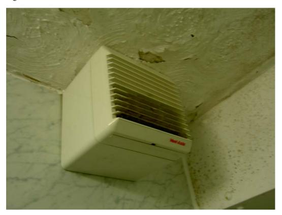
Figure 6.3c—Vent duct connected to outside
